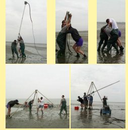
Fig. 2: The sediment cores were taken by a vibrocorer and recovered by a lifting block.
